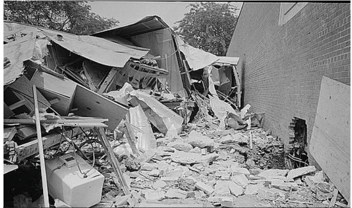
Bomb damage at the Gaston Motel
